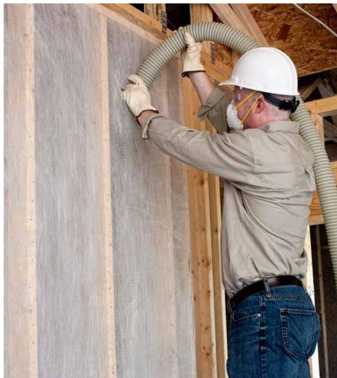
4. A small machine capable of blowing 1800 pounds of GreenFiber Loose-Fill Insulation per hour should have the gate open approximately 50% and the air pressure set at two-thirds open. As machine capacity increases, the gate should be reduced and the air pressure turned down.
